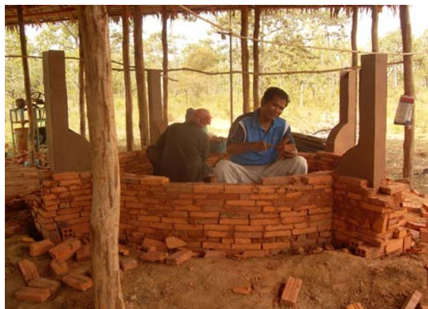
Picture 10: Construction of improved charcoal kiln, Pursat
